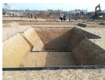
(a) Slope excavation
