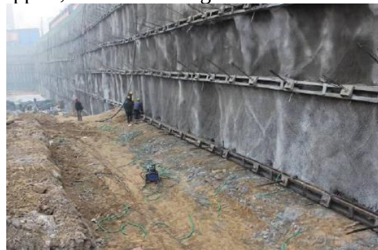
(b) Pile + anchor support
