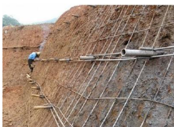
(b) Soil nailing support
