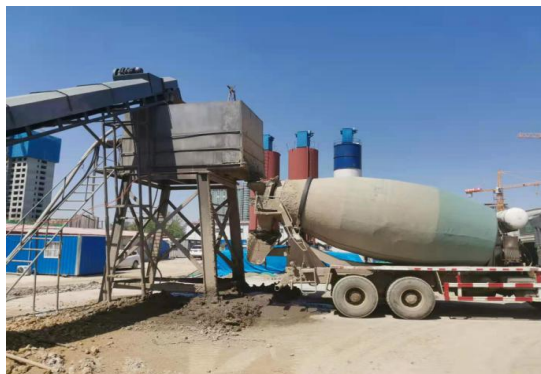
Figure 5. Transportation of high-early-strength soil cement
