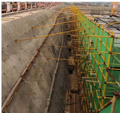
Figure 1. Space of the foundation trench
