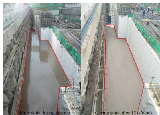
Figure 6. Flowing state during casting and hardening states after casting
