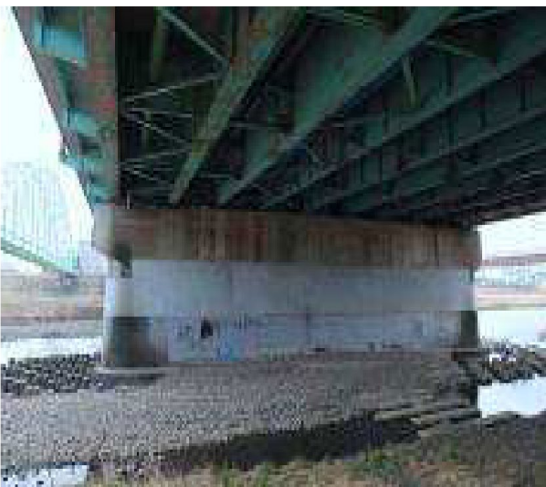
Figure 4. Sendai Bridge and its bearing [8]
