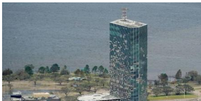
Figure 8. The damage to the glass curtain wall during the hurricane happened in Lake Charles, Louisiana
