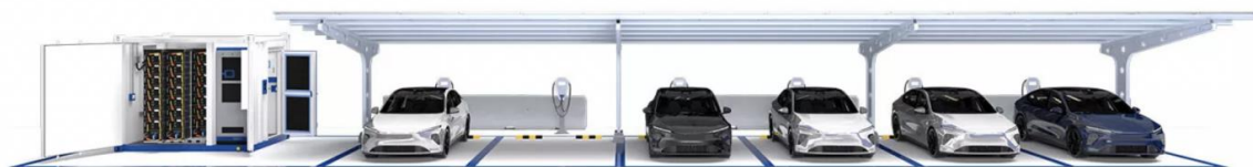
Fig 5. Photovoltaic–energy storage charging station.
