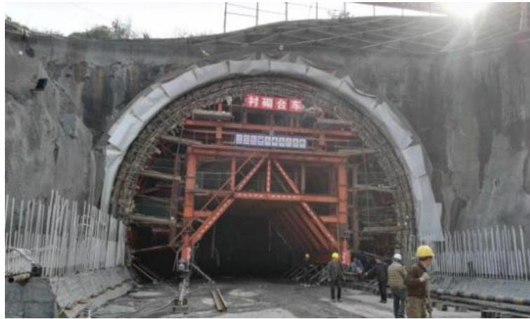
Figure 1. Tunnel entrance section.
