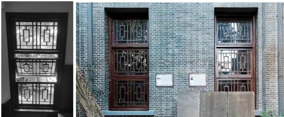
Fig. 15 Sicheng Hall clear water brick wall and supporting window.
