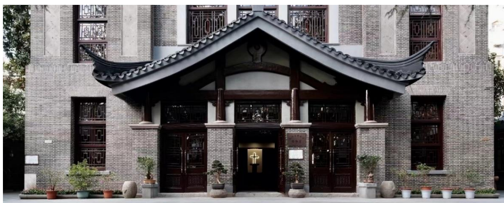
Fig. 13 Sicheng Hall roof and cornice.
