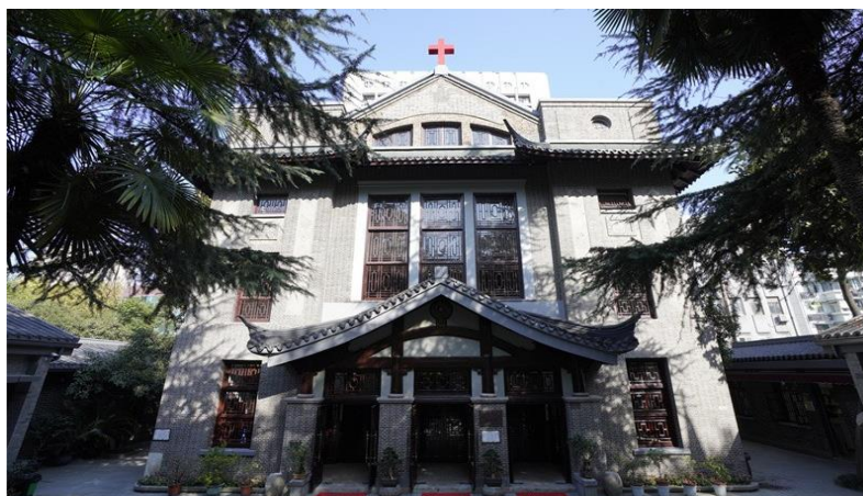
Fig. 12 The facade of Sicheng Hall.
