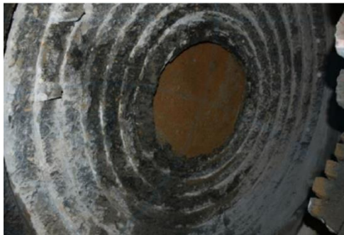
Fig 13. Breaking the main tunnel door.
