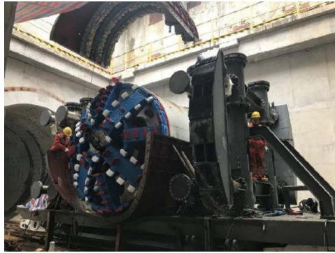
Fig 12. TBM assembling in launching shaft.
