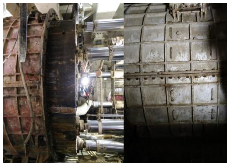
Fig 6. Sleeve for Mirco TBM launching and receiving.
