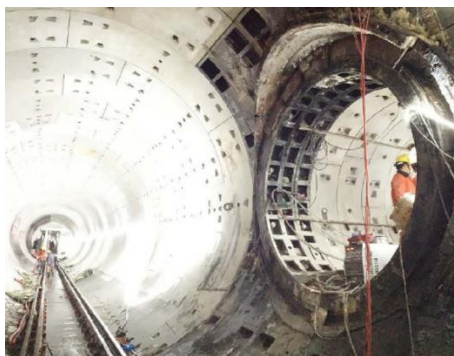
Fig 14. Formed connecting passage.
