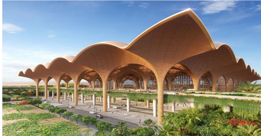
Figure 1. Overall Effect of Cambodia's New Phnom Penh Airport Project
