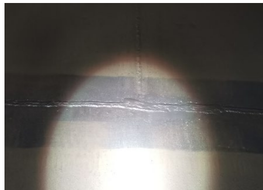
Figure 6. Weld area after surface treatment of weld inspections
