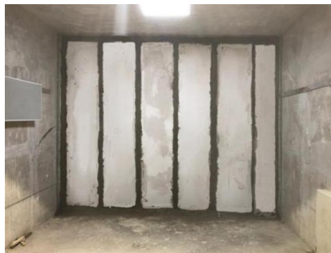
Figure 6. Installation of wallboard for sound insulation experiment
