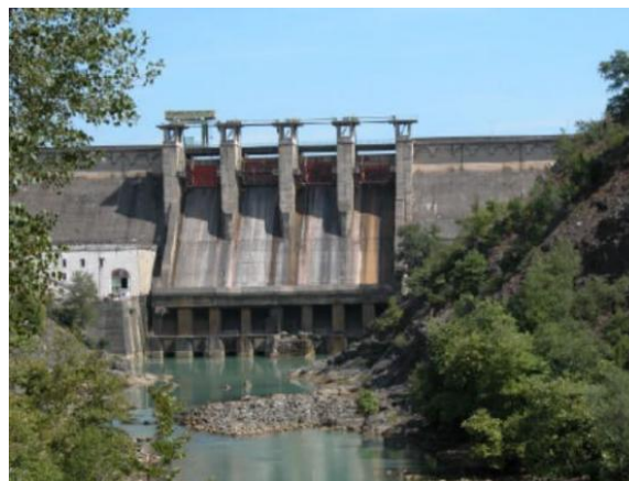
Figure 4. Construction of Spillway Using HPC
