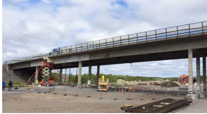
Figure 2. HPC Used in Flyover Construction
