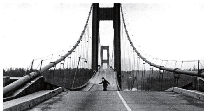
Fig 1. Twisty sponge bridge, Tacoma Narrows Bridge [6].
