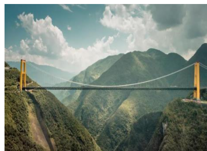
Fig. 2 Bridge across the valley
