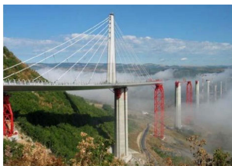
Figure 11. Construction of the deck and the pylons
