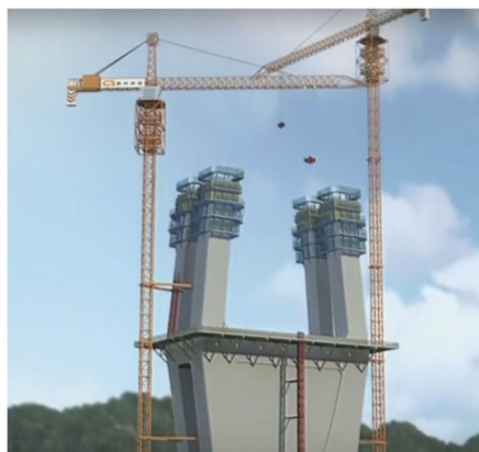
Figure 5. Demonstration of mould climbing techniques
