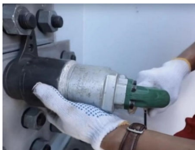
Figure 8. Workers on site tighten high-strength bolts
