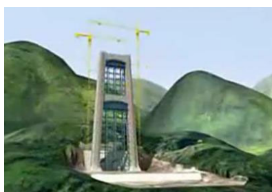
Figure 4. Erection of the bridge tower
