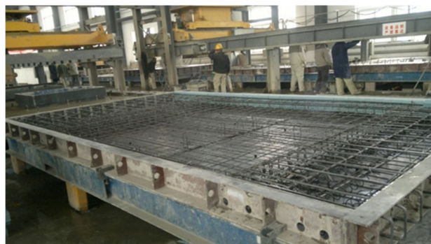
Figure 2. Production site of prefabricated slabs
