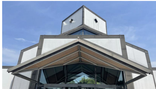
Fig. 3. Exterior Roof Structure
