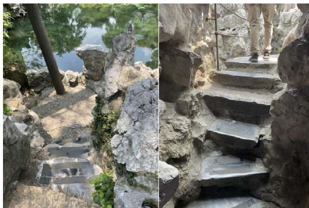
Figure 6. Anti-slip tape on rockeries
