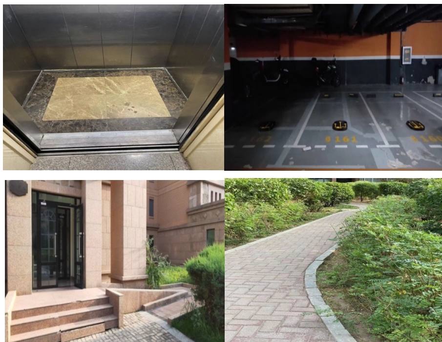
Figure 1. Elevators, parking spaces, ramps, and walkway facilities in the community
