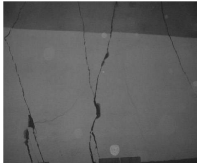
Fig. 1 dislocation of tunnel lining Fig. 2 cracking of lining Fig. 3 spalling of lining
