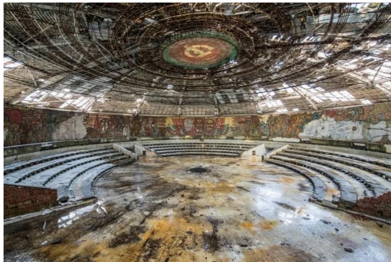
Figure 3. Auditorium of Buludazha monument.
