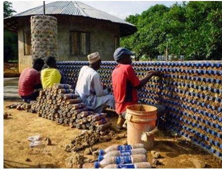
Fig. 3 Workers laying plastic bottle bricks for The Bottle House [10]
