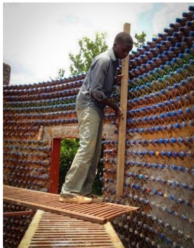
Fig. 4 Settings of plastic bottle bricks for the Bottle House [10]
