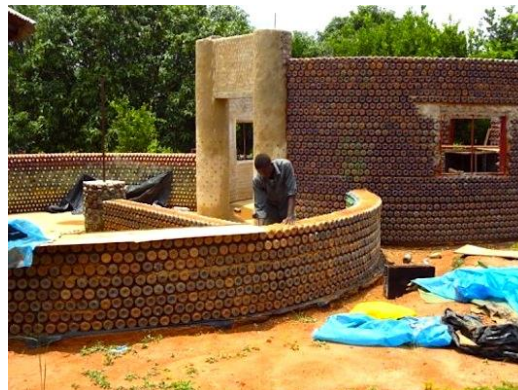
Fig. 5 Workers plastering the wall of the Bottle House [10]
