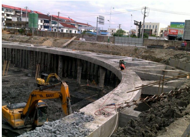
Figure 1. Construction process of deep foundation pit engineering
