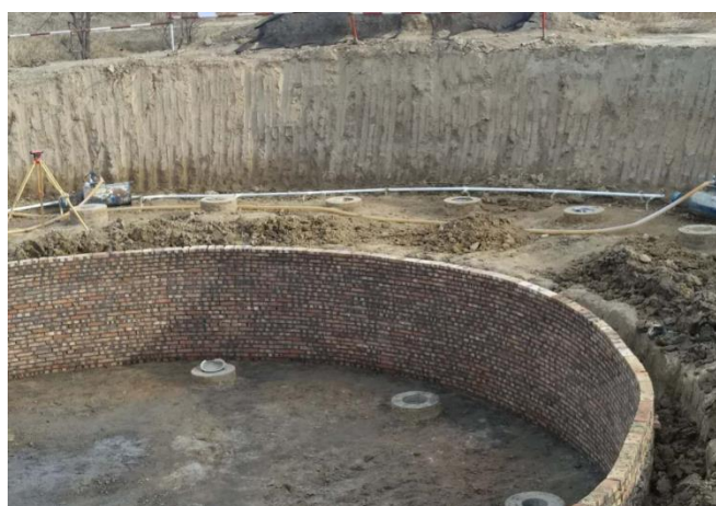
Figure 2. Groundwater control in foundation pit construction
