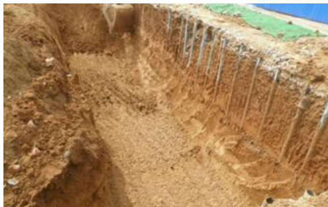
Figure 1 Foundation pit supporting structure
