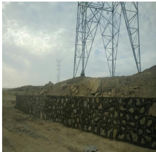
Figure 4: Flood control dam
