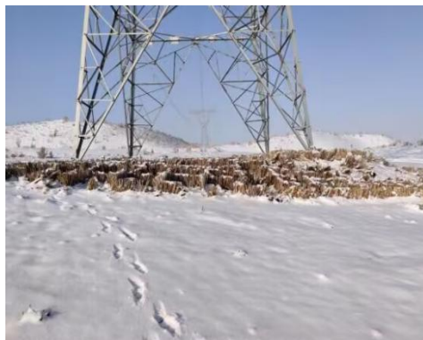
Fig. 2: Grass checkerboard for wind prevention and sand fixation
