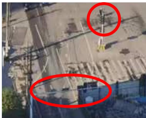
Figure 2. The signal lights are not arranged reasonably
