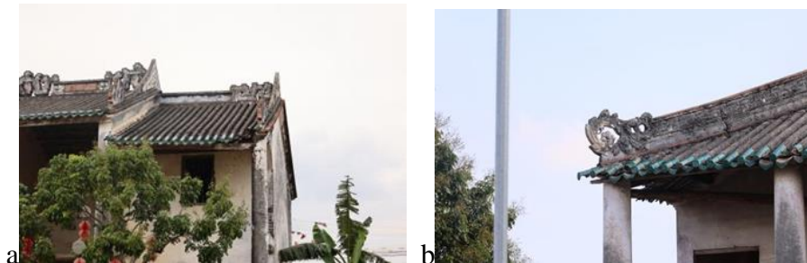
Fig. 5. (a) North door ridge and cornice pattern; (b) South Gate cornice pattern
