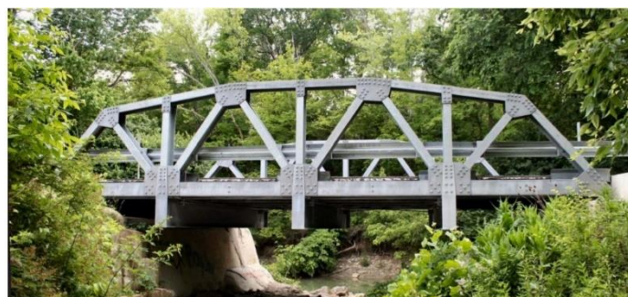
Fig. 1 Pony Truss Bridge [10]
