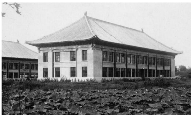
Fig. 7 Roof of Yenching University building
