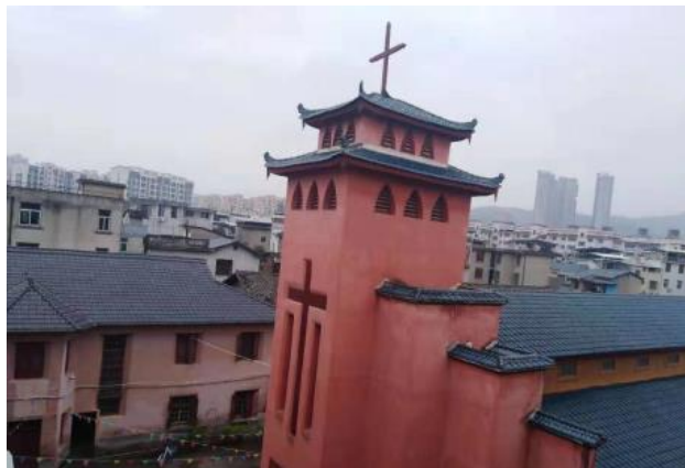
Fig. 3 Rammed earth wall of Changting Catholic Church
