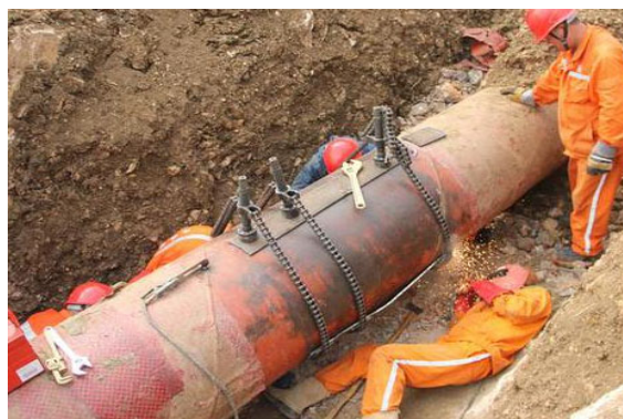
Figure 8. Welding plate reinforcement
