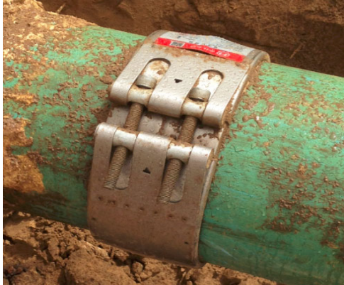
Figure 11. Mechanical clamp reinforcement
