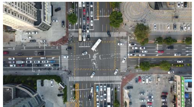
Figure 2. Intersection of North New Road and College Road
