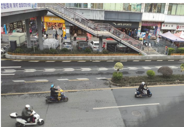
Fig 1. Non-motorized vehicles illegally entering motor vehicle lanes.
