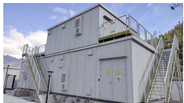
Figure 2. On-site view of the prefabricated modules
