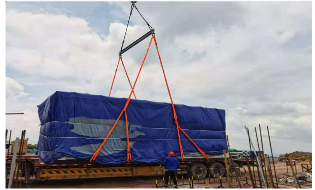
Figure 1. Lifting diagram for a prefabricated module measuring 10,200×3,050×3,950 mm
