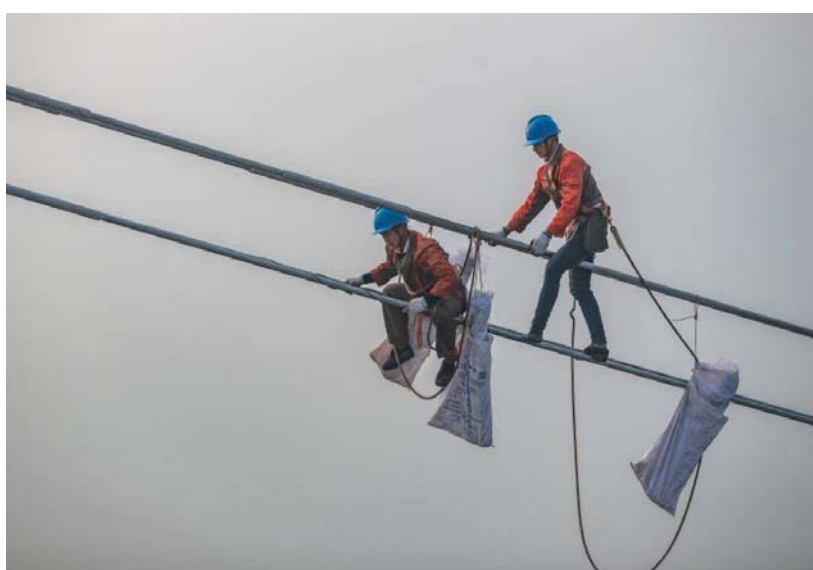
Figure 1. Transmission line stringing process
