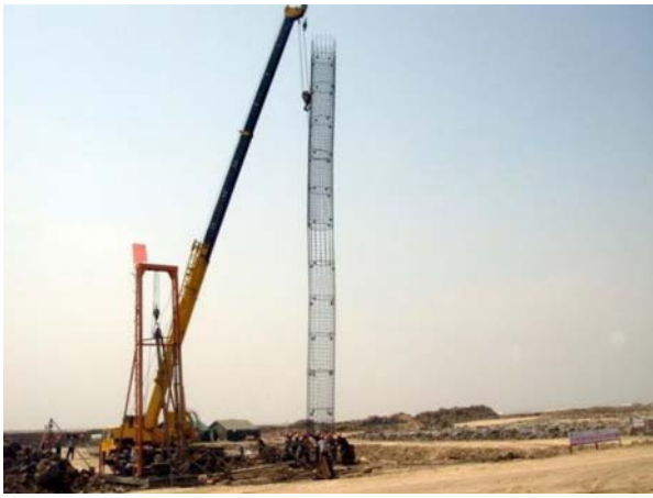
Figure 1. Construction process of cast-in-place pile for transmission line in plateau
