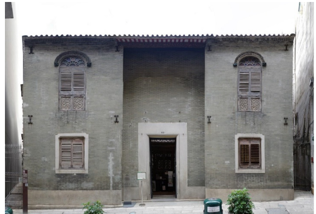
Fig 1. Front view of Lu's house
