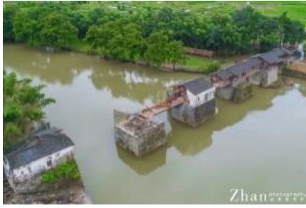
Fig 6. Rainbow Bridge after washout
