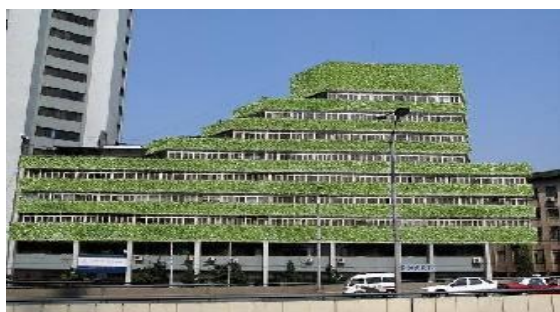
Figure 1. Greening of the wall
