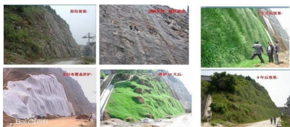
Figure 3. Greening of slopes
