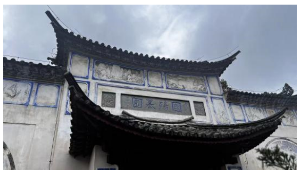
Figure 5. Tengchong Traditional Residential Settlement
