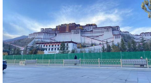
Figure 4. The use of red and white on the façade of the Brada Palacer
