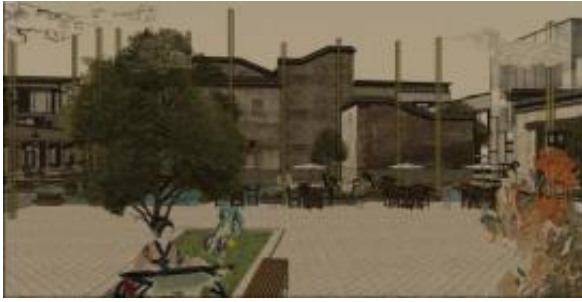
Figure 5. Building facade renovation
