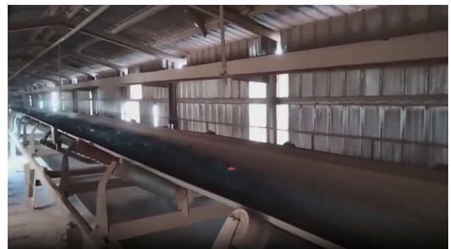
Figure 4. Field application photos
