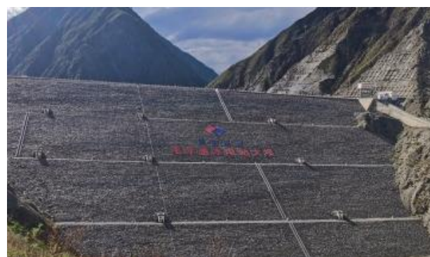
Fig.2 Photos of on-site investigation in Heishui County
